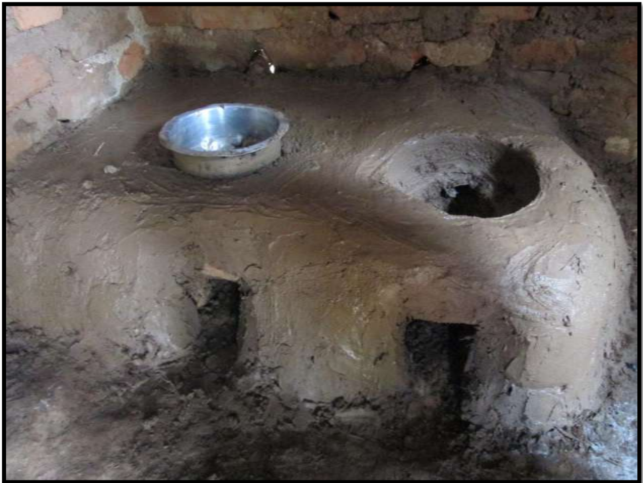
Figure 7: Double Rocket Stove with 2 Chimneys to direct smoke out of the kitchen. Made by the Permaculture students.
